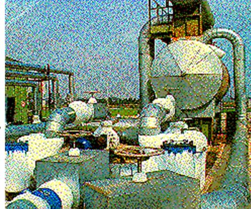
The 44 freeze pipe holes, with 127mm diameter casing, were drilled on a 22m diameter circle, and the freeze was [computer-monitored](#). A central drill hole formed a pressure relief drain for groundwater expelled within the constricting ice front.
