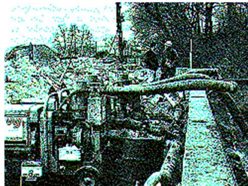
unnecessary in this area, so the wellpoints were installed along the bank of the stream at the east boundary, and around the southern boundary. Groundwater in that area is almost at surface level.
