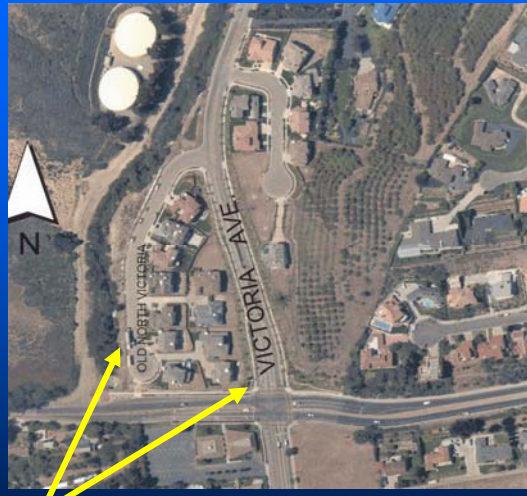
Roadway realigned as part of mitigation for residential tract
