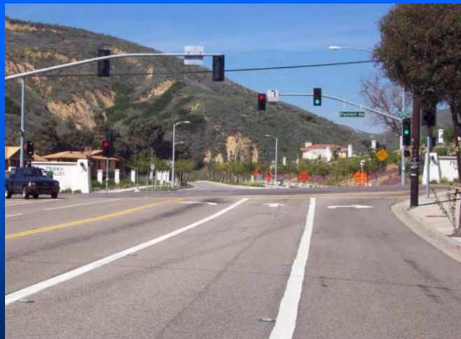
Roadway realigned as part of mitigation for residential tract
