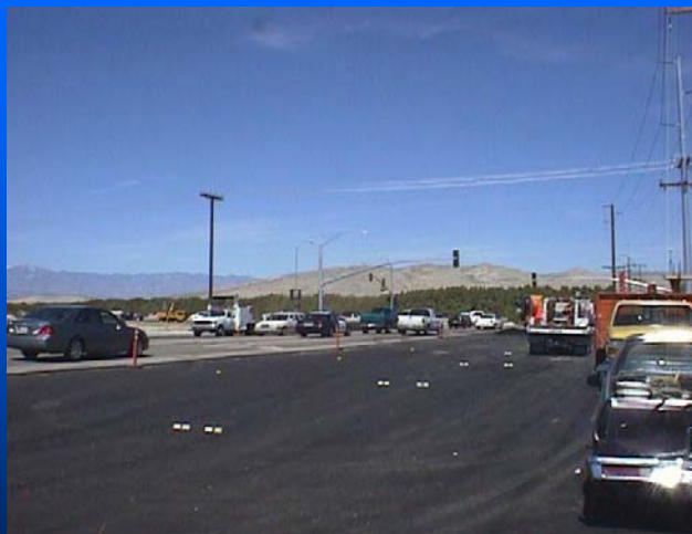
Closest impacted intersection widened and signalized as part of mitigation measures
