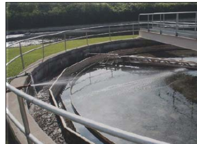
Trickling filter
