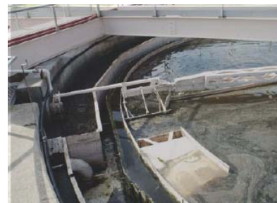
Secondary sedimentation tank and clarifiers
