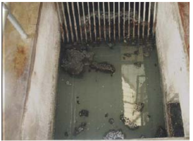
Coarse solids removal rack/screen
