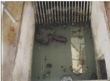
Coarse solids removal rack/screen
