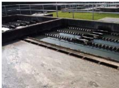
Primary sedimentation tank and clarifiers
