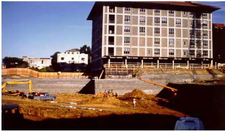
Figure 7 - North West Animal Facility, University of California at Berkeley
