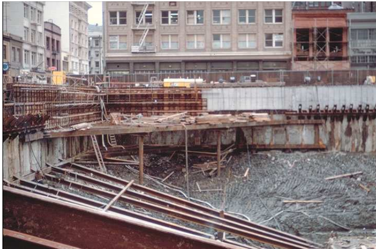
Figure 13 - Raker bracing for wide excavations
