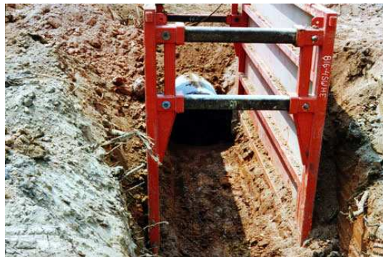
Figure 2 – A typical trench box
