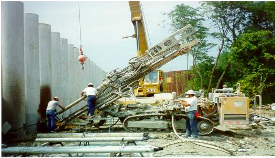
Figure 15 - Tieback being installed
