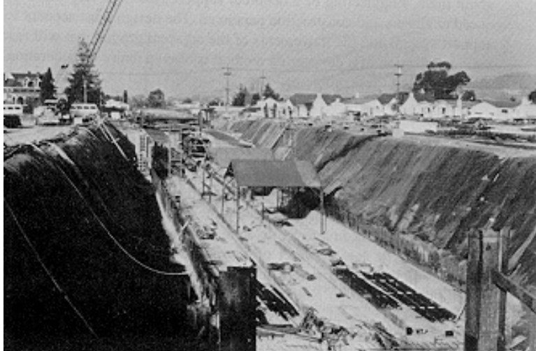
Figure 1b - Use of plastic sheets for slope protection in a shallow excavation
