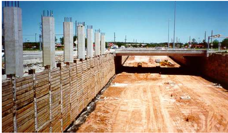
Figure 5 - Two examples of soldier beams and lagging method used for retaining walls
