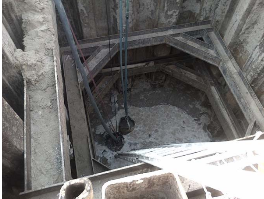
FIGURE 2-3 UNCONTROLLED DEWATERING FROM A SUMP WITHIN A SHORED PIT, SHAKHOUT CITY, 2013
