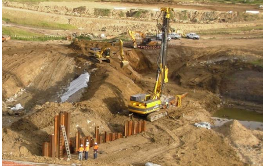
FIGURE 8-1 TYPICAL SHEET PILE CUTOFF DURING CONSTRUCTION
