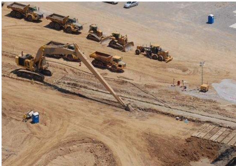
FIGURE 8-3 LONG REACH EXCAVATOR
