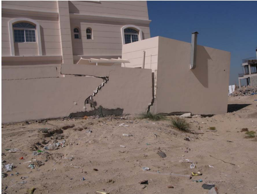
FIGURE 2-11 TILTING OF GRADE SUPPORTED GUARD ROOM IN KHALIFA CITY, SECTOR SW-12
