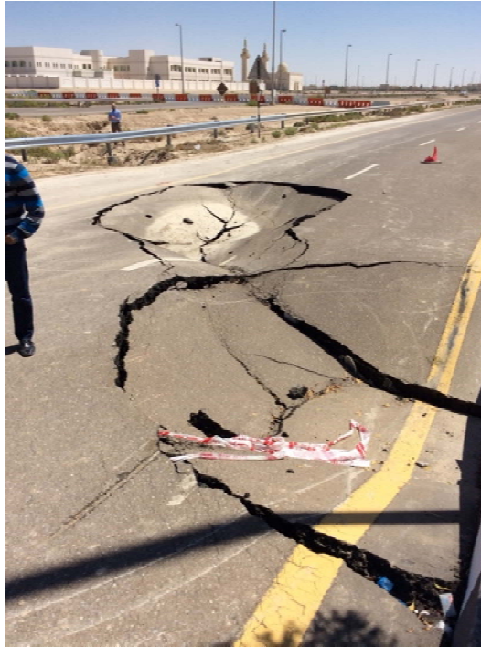
FIGURE 2-16 COLLAPSE OF INTERNAL ROADS IN SHAMKHA, SECTOR SH-13, IN MARCH 2014 DUE TO EROSION OF ROAD SUBGRADE AND LOOSE UNDERLYING LAYERS FOLLOWING HEAVY RAINSTORMS
