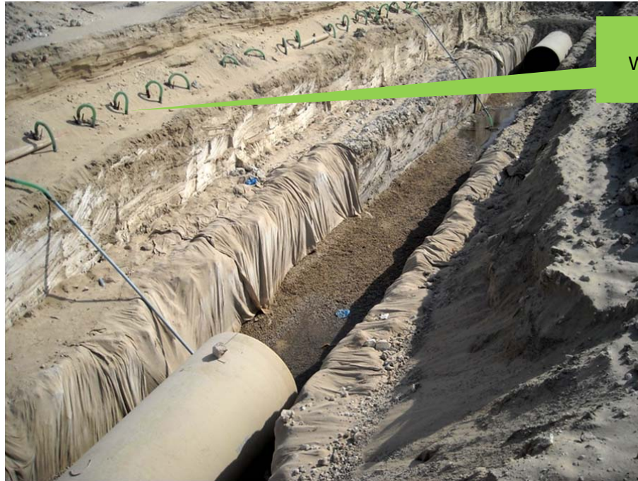
FIGURE 2-5 WELL POINTS DEWATERING SYSTEM FOR AN INFRASTRUCTURE UTILITY LINE IN KHALIFA CITY, 2010
