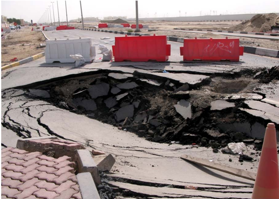
FIGURE 2-7 CLOSE UP OF FAILURE SHOWN ON FIGURE 2-6
