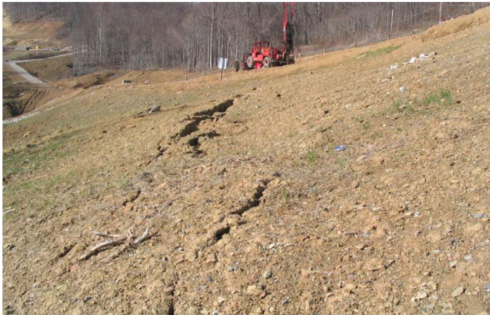
FIGURE 6-1 CRACKING DUE TO SLOPE INSTABILITY
