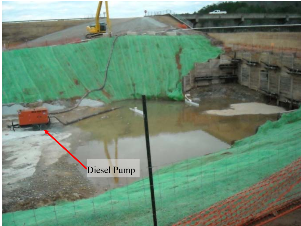
FIGURE 4-2 DEWATERING BY SURFACE PUMPING
