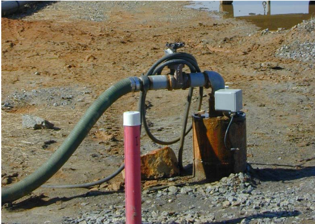
FIGURE 4-12 TYPICAL DEWATERING WELL
