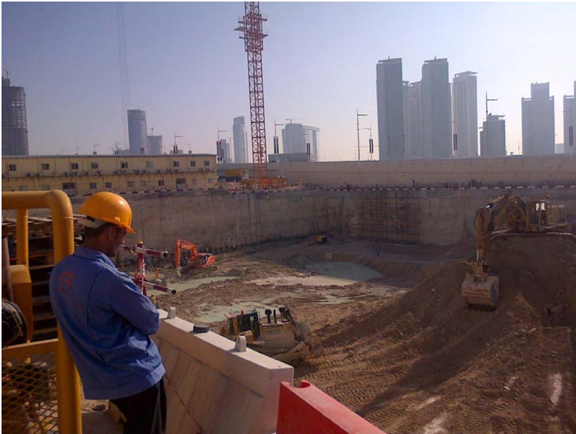
FIGURE 4-3 DEWATERING BY SURFACE PUMPING IN A DEEP SHORED EXCAVATION IN ABU DHABI CITY
