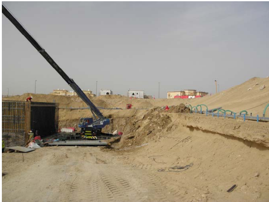
FIGURE 2-4 WELL POINTS DEWATERING SYSTEM IN SHAKHOUT CITY, 2011
