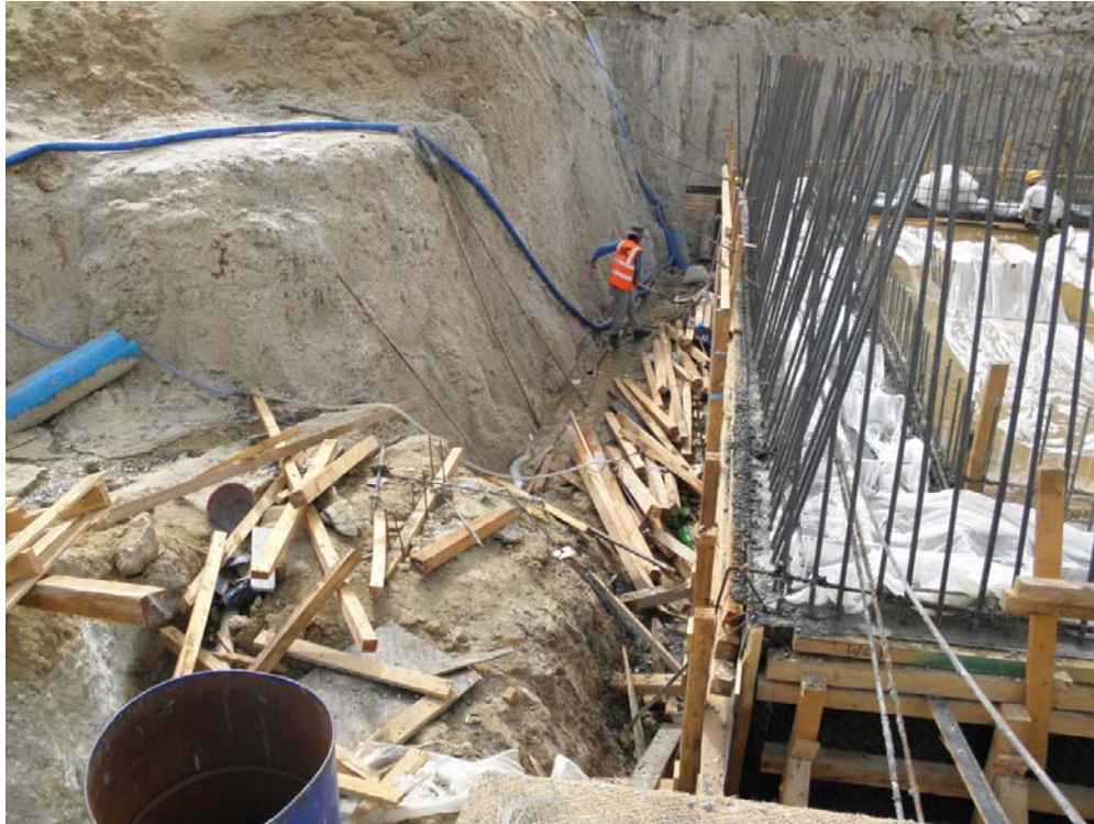
FIGURE 4-4 UNCONTROLLED DEWATERING BY OPEN SUMP IN A DEEP EXCAVATION IN SHAKHBOUT CITY, 2011
