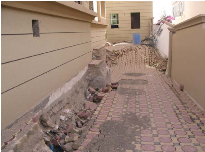
FIGURE 2-8 GROUND FAILURE IN A RESIDENTIAL PLOT IN KHALIFA CITY SECTOR SW-12 ATTRIBUTED TO NEARBY UNCONTROLLED DEWATERING, 2010
