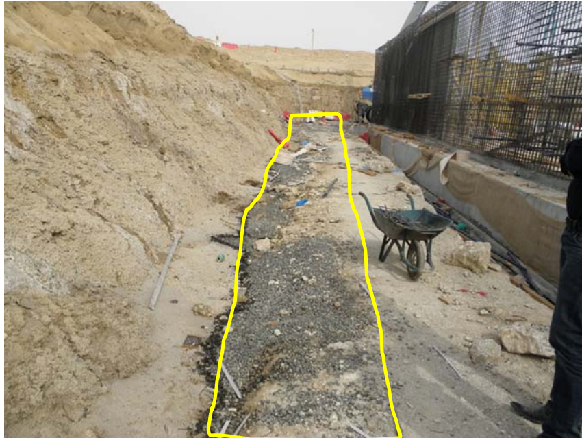
FIGURE 4-6 TOP OF A FRENCH DRAIN FOR DEWATERING OF A DEEP EXCAVATION IN SHAKHBOUT CITY, 2011
