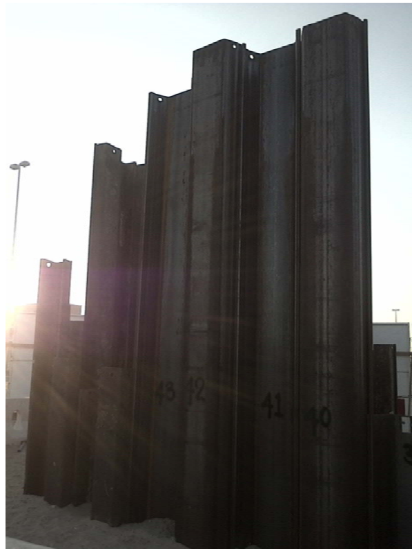
FIGURE 8-2 SHEET PILE CUTOFF FOR CONSTRUCTION OF DRIVING PIT IN SHAKHBOUT CITY, 2013
