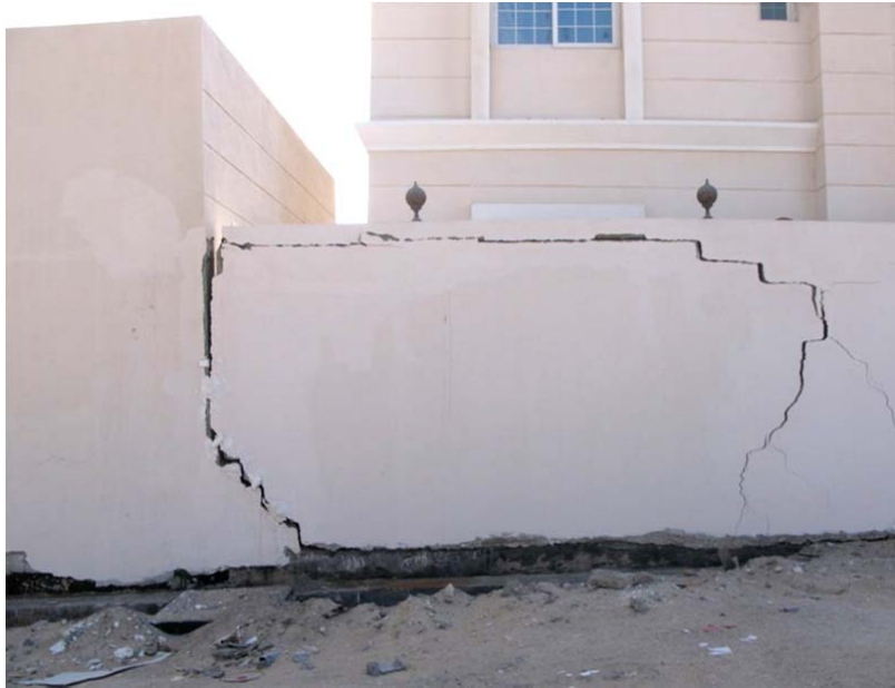
FIGURE 2-9 DAMAGE TO SHALLOW SUPPORTED BOUNDARY WALL IN KHALIFA CITY SECTOR SW-12 DUE TO GROUND SETTLEMENT ATTRIBUTED TO A NEARBY UNCONTROLLED DEWATERING, 2010
