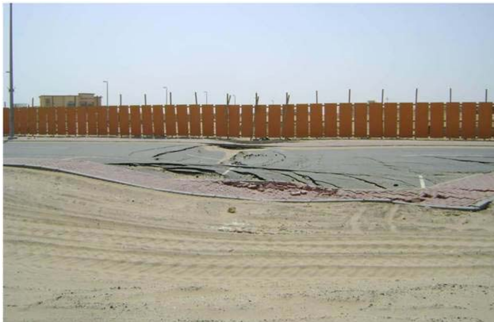
FIGURE 2-12 COLLAPSE OF ROAD 5 AND ADJACENT PLOT IN SHAKHBOUT CITY CAUSED BY ADJACENT UNCONTROLLED DEWATERING ACTIVITIES, 2011
