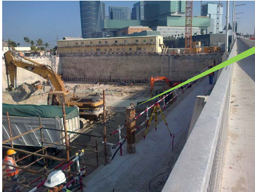
FIGURE 2-1 DEEP WELL INSTALLED IN THE DIAPHRAGM WALL OF A DEEP EXCAVATION IN ABU DHABI ISLAND, 2014
