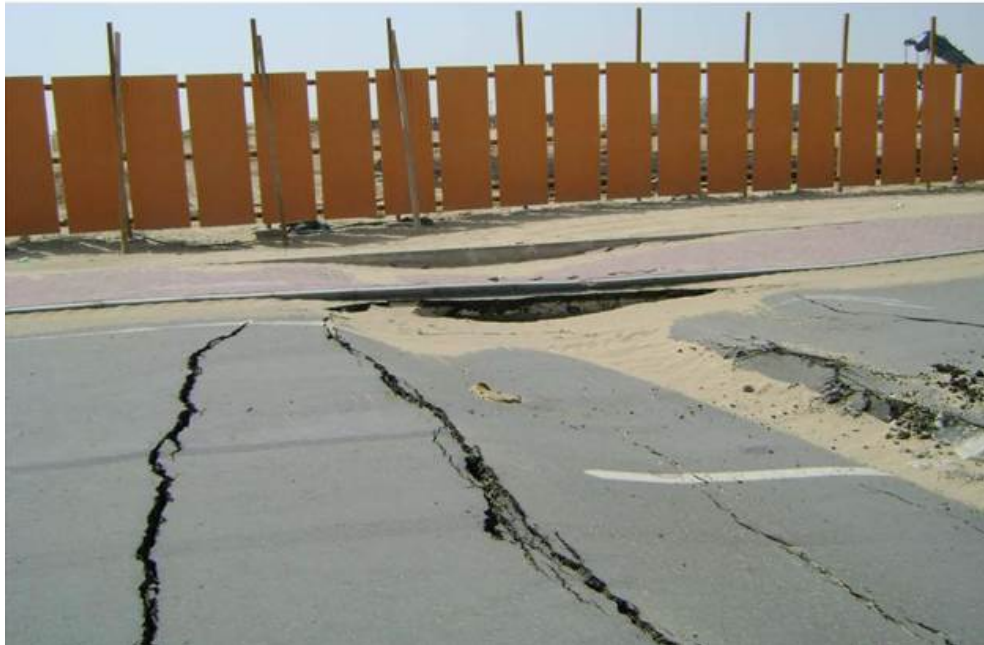
FIGURE 2-13 COLLAPSE OF ROAD 5 AND ADJACENT PLOT FROM UNCONTROLLED DEWATERING ACTIVITIES
