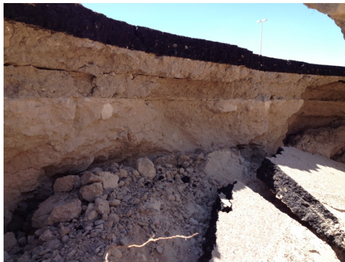
FIGURE 2-17 EXPOSED ROAD BASE, SUBBASE, AND UNDERLYING LOOSE LAYERS OF A COLLAPSED SECTION OF AN INTERNAL ROAD IN SHAMKHA, SECTOR SH-13, MARCH 2013
