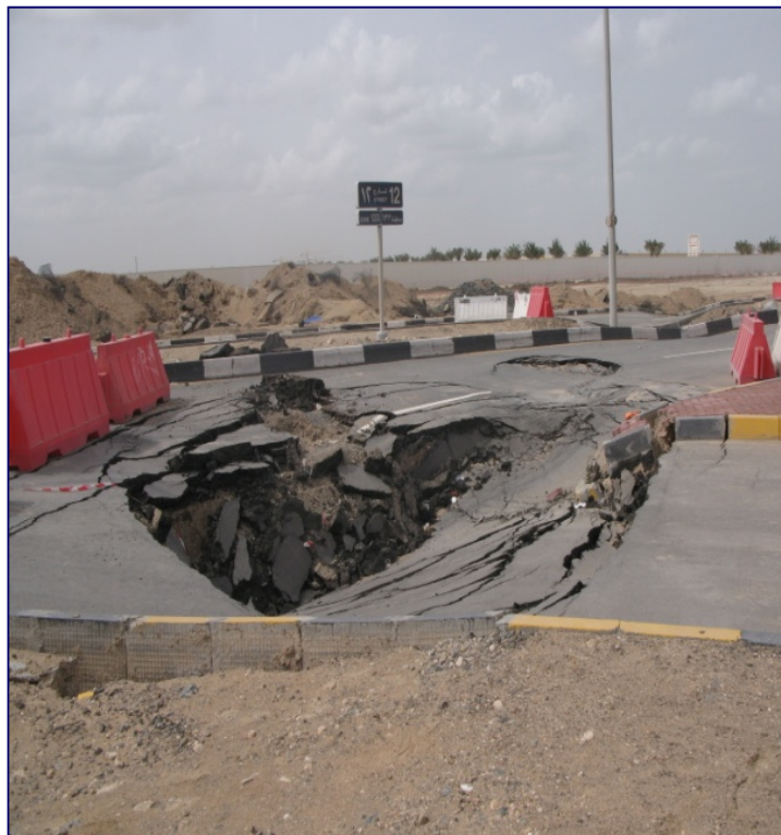
FIGURE 2-6 FAILURE IN AN INTERNAL ROAD IN KHALIFA CITY SECTOR SW-12 ATTRIBUTED TO NEARBY DEWATERING
