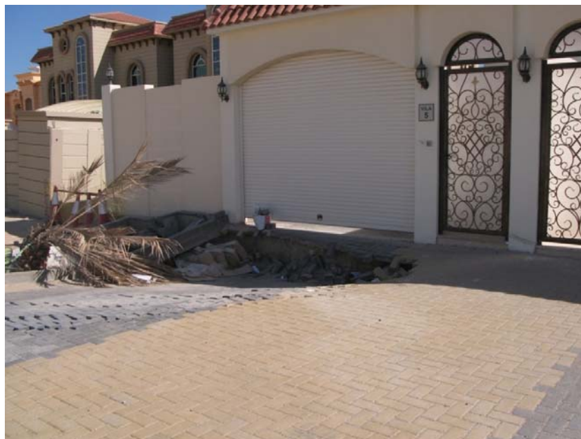
FIGURE 2-10 GROUND FAILURE IN THE SIDEWALK OF A RESIDENTIAL PLOT IN KHALIFA CITY, SECTOR SW-12, ATTRIBUTED TO A NEARBY UNCONTROLLED DEWATERING, 2010
