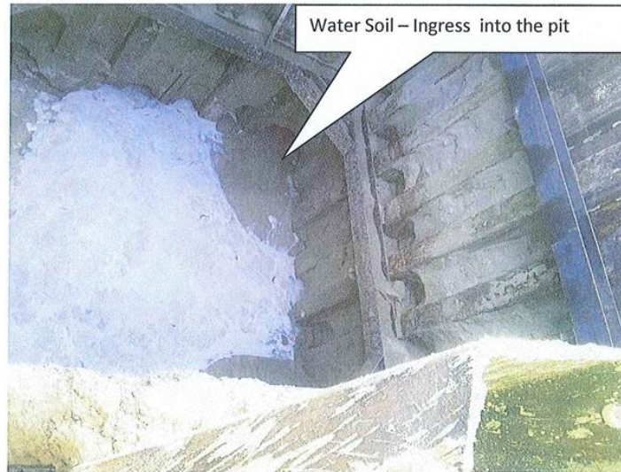
FIGURE 2-14 WATER-SOIL INGRESS INTO THE PIT OF A SHORED EXCAVATION DUE TO POOR INTERLOCKING OF SHEET PILES, SHAKHBOUT CITY, 2013
