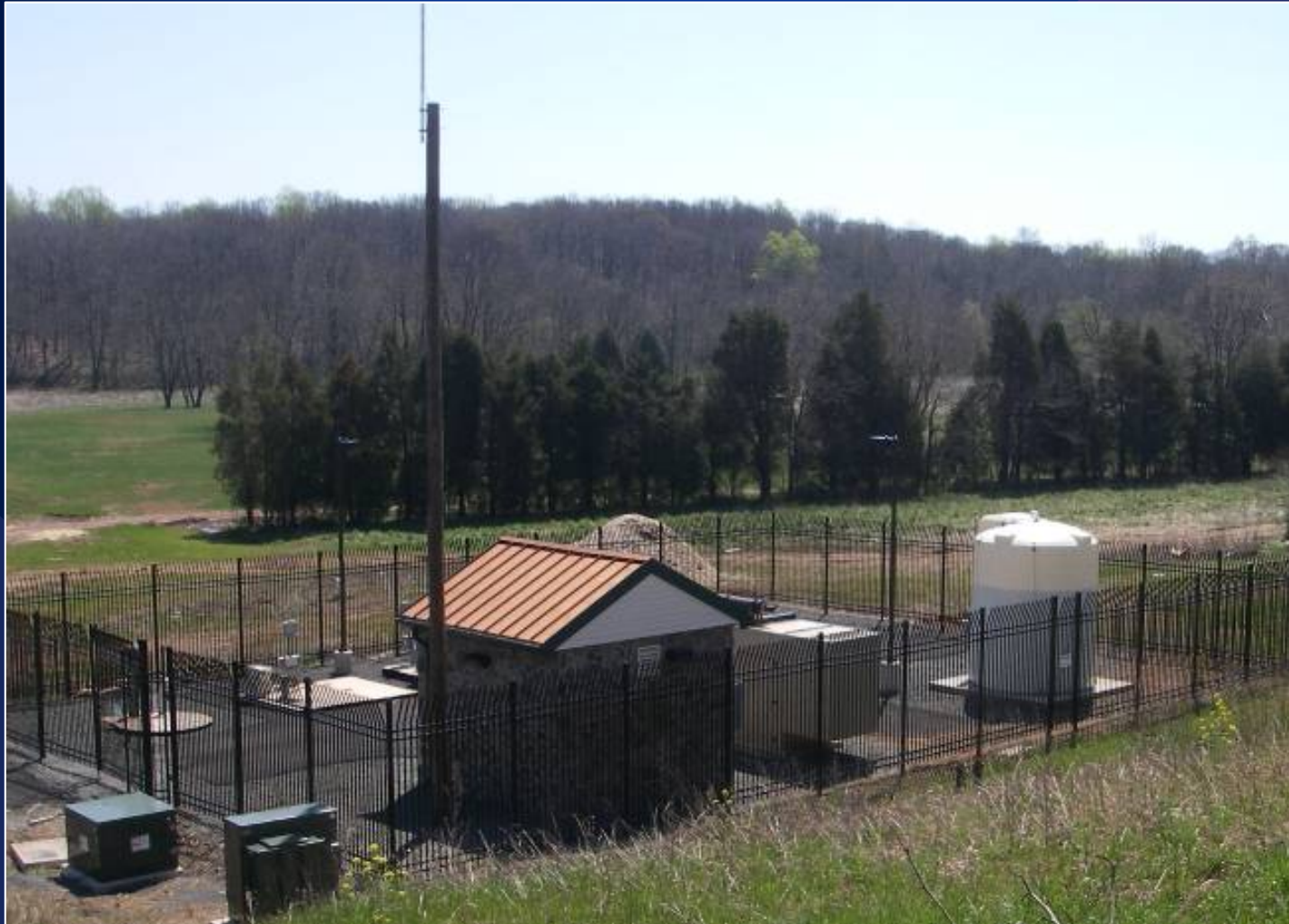
Prince William County Service Authority Morris Farm Pump Station 928 GPM Capacity
