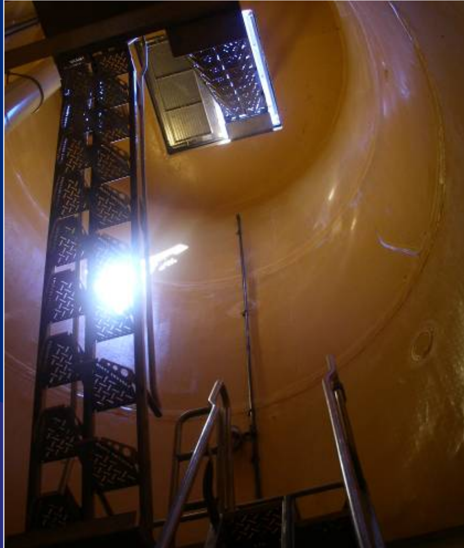
Prince William County Service Authority Morris Farm Pump Station Grinder Vault with HPDE Liner & Stainless Steel Stairs
