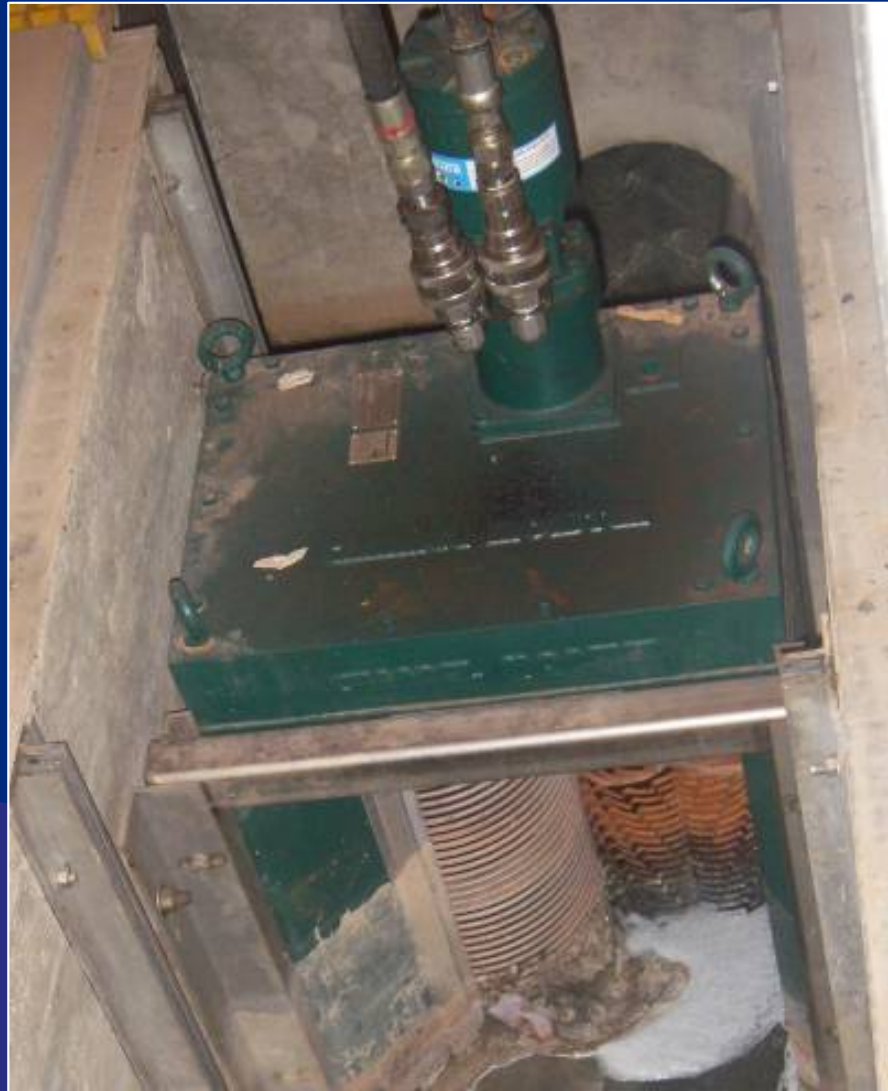
Prince William County Service Authority Morris Farm Pump Station Grinder
