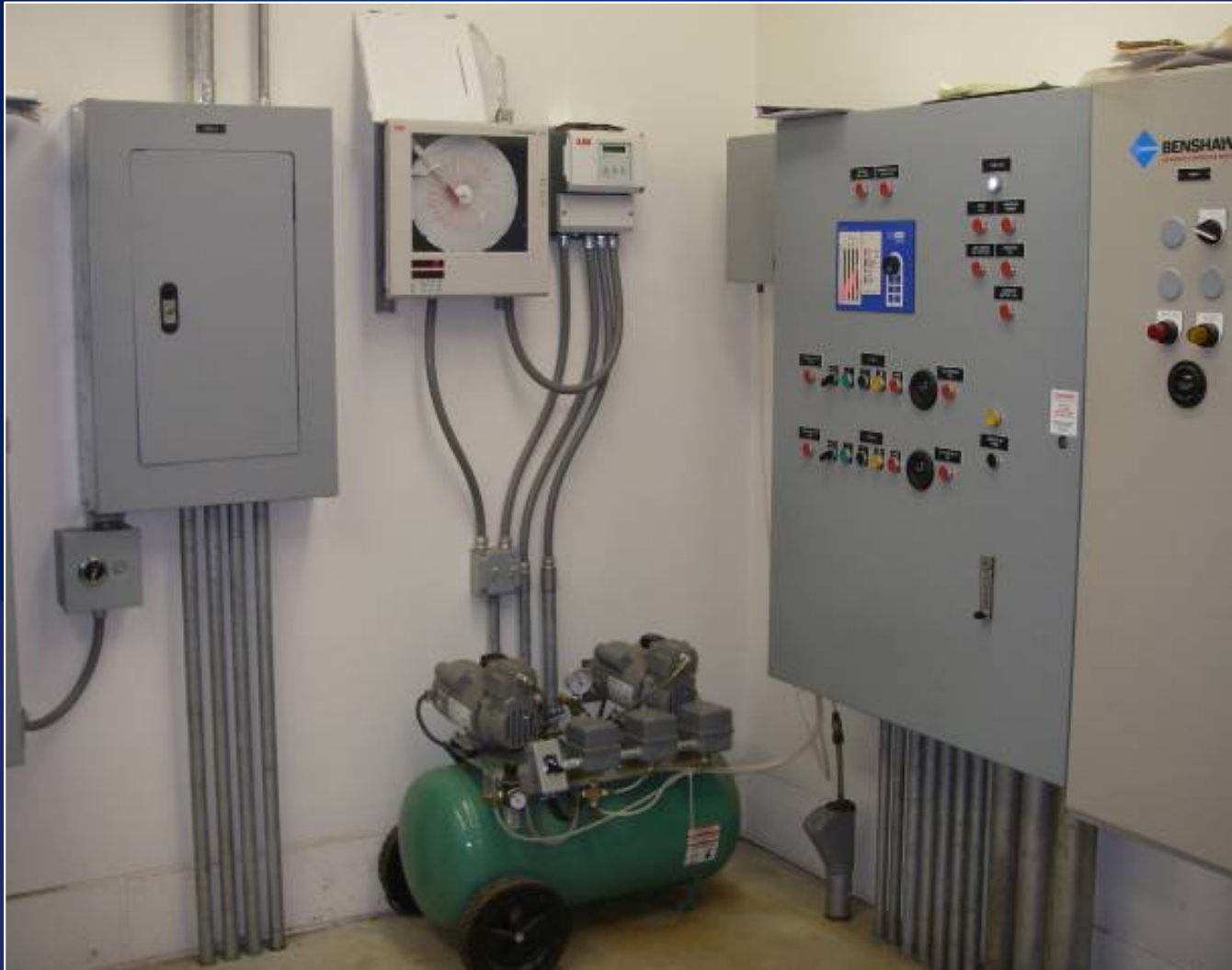
Prince William County Service Authority Morris Farm Pump Station Control Building Panels
