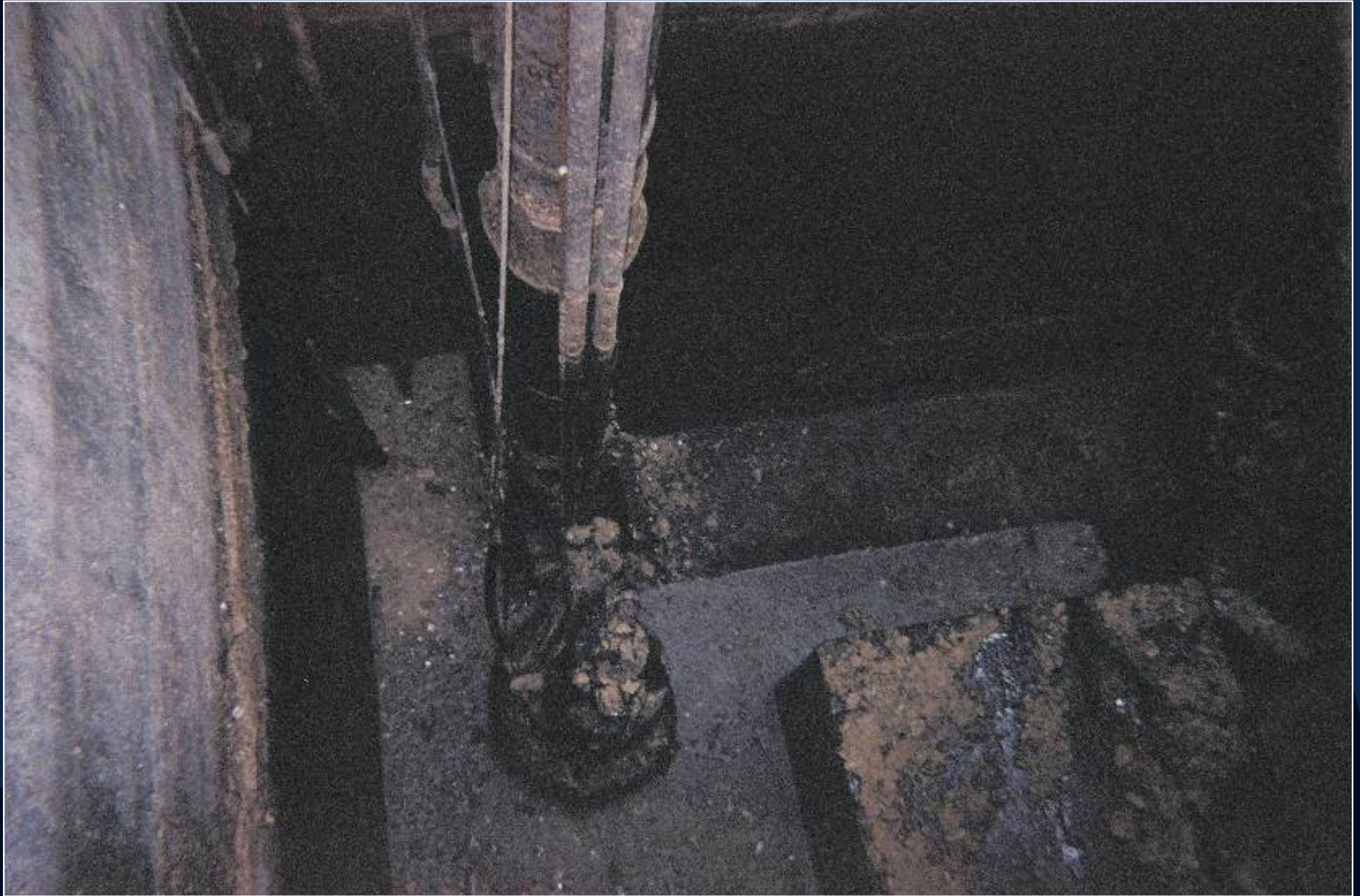
100 MGD Pump Station
