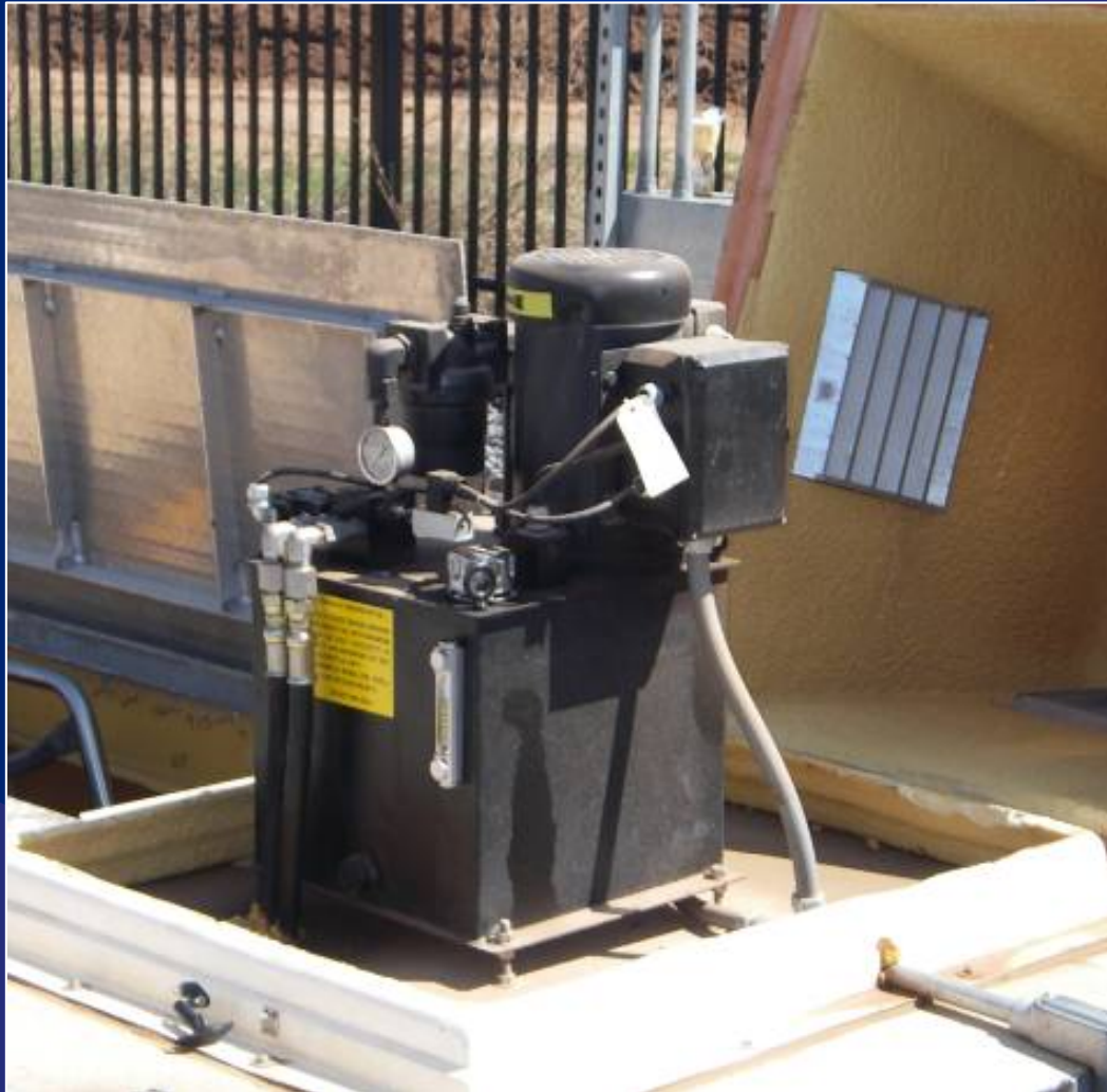
Prince William County Service Authority Morris Farm Pump Station Grinder Hydraulic Power Drive
